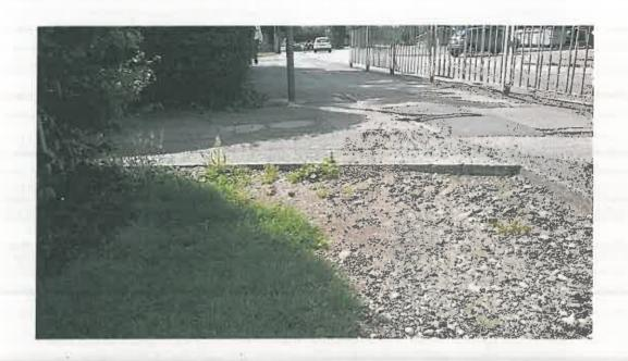
Photo No. 3. - View of South End of Verge Showing Degree of Setlement Within Verge.
