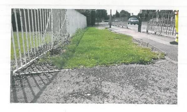
Photo No. 2. - View North End of Verge Showing missing and Uneven Edge Stones
